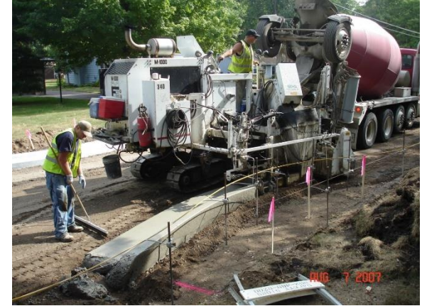
Curb & Gutter Installation
