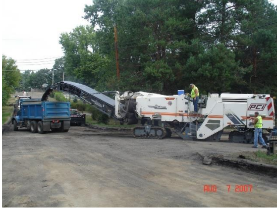
Removing Pavement
