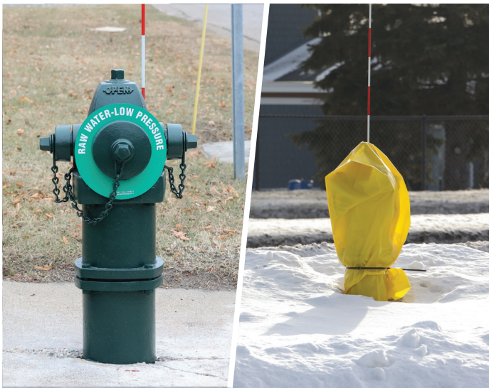
"Raw water" hydrants have been painted olive green, while regular hydrants along high-traffic roadways have been plastic wrapped for winter.
